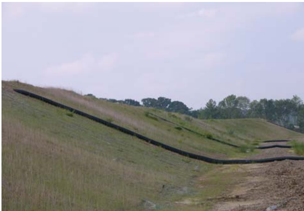
Figure 2. Diagonally Placed Downdrain
