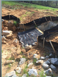
An approved Silt Fence has not been attached to the structure
