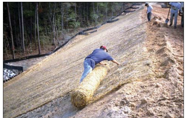
Figure 2. Installation of Jute Matting
