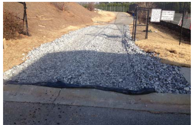
Figure 2. Geotextile Underliner
