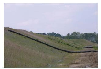
Figure 2. Diagonally Placed Downdrain
