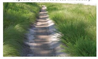
Figure 1. Concrete Lining
