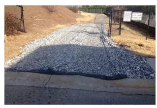
Figure 2. Geotextile Underliner
