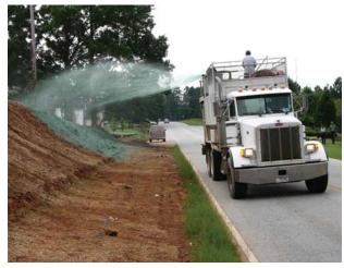
Figure 1. Hydroseeding on disturbed areas
