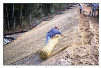
Figure 2. Installation of Jute Matting
