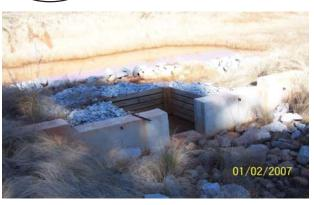
Figure 3. Slotted Board Dam
