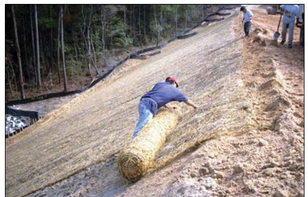
Figure 2. Installation of Jute Matting
