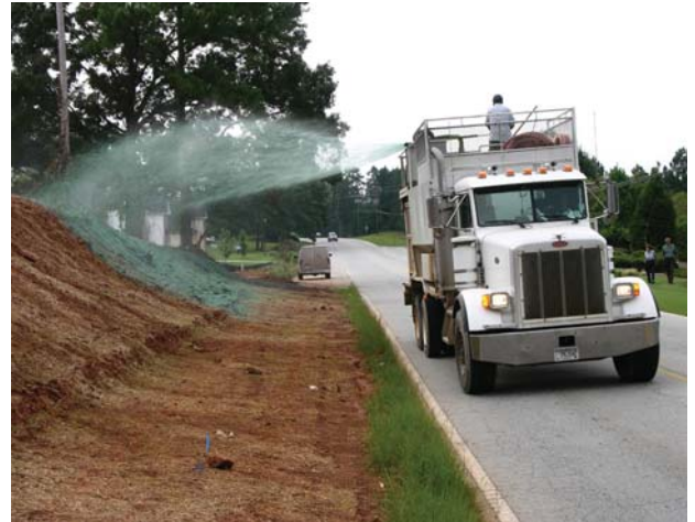
Figure 1. Hydroseeding on disturbed areas
