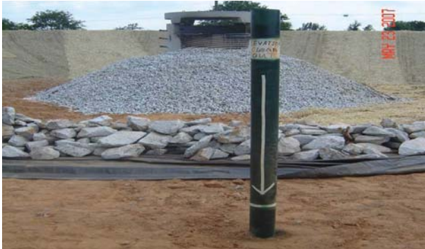
Figure 5. Clean-out marker
